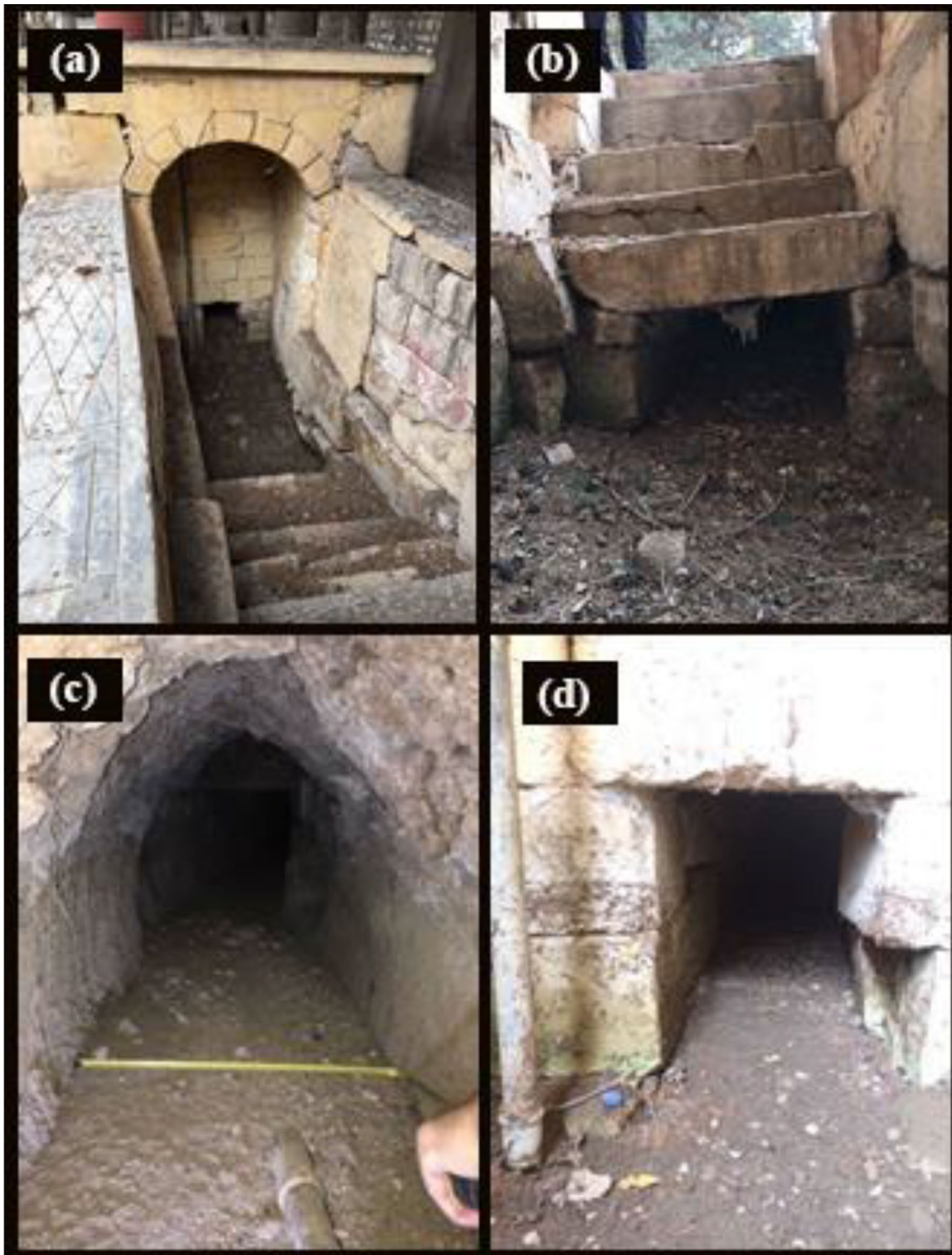
Fig. 8 The details of karez galleries of Little and Middle Springs of Germuş Water; a-d. Views of Circular Galleries and Stone Braid Walls of Tunnels, from Site Study of the Authors
