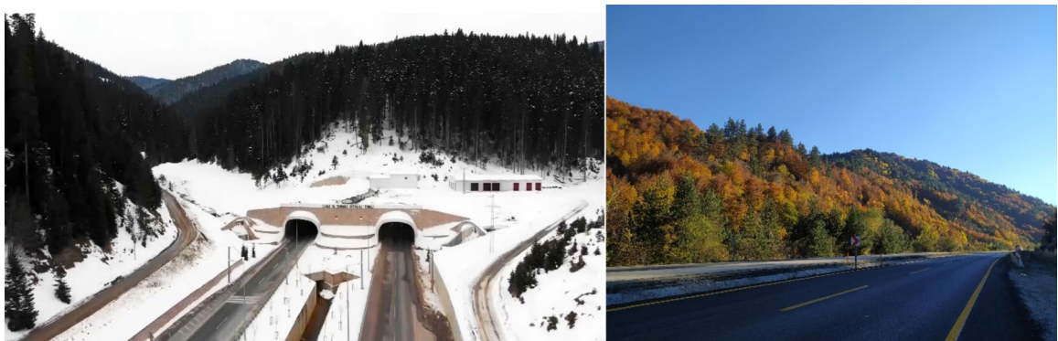
Fig. 2 Photo of Ilgaz Mountain Highway Tunnel and Old Forest Road
